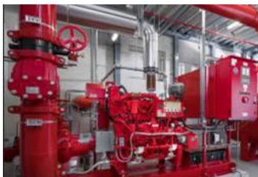
Fire Pumps Set of 1250 capacity
